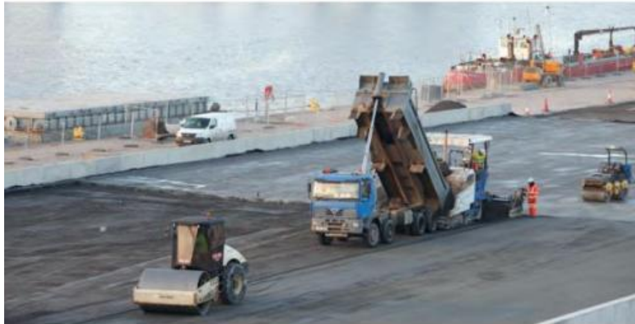
Figure 3. RCC roadway construction in the UK using RCC
