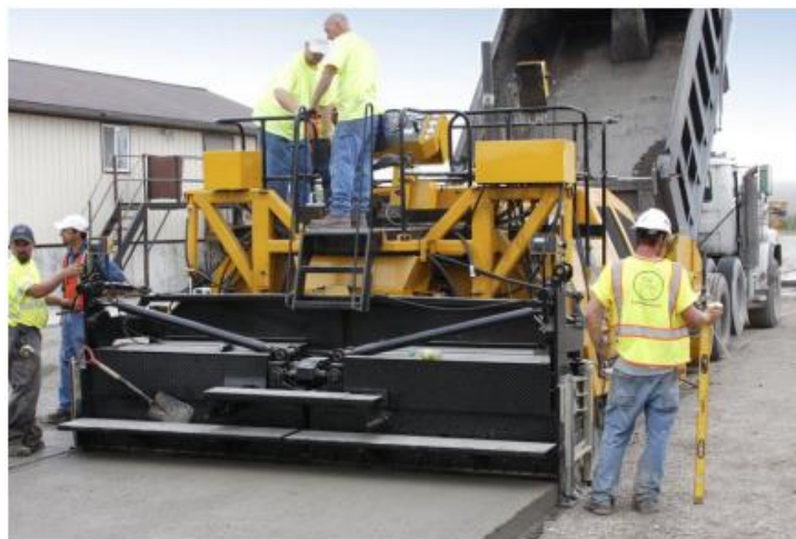
Figure 2. Roller-compacted concrete (RCC) placement
