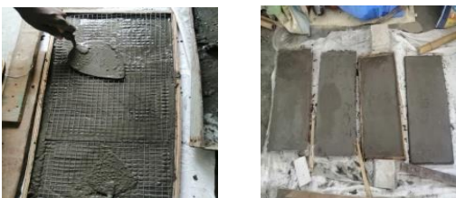
Fig 2 - Casting of ferrocement panel
