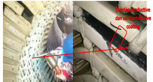
Figure 3.10 Application of varnish in corona protection semi conductive coating
