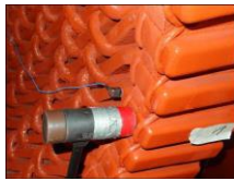
Figure 3.1 Bump Test End Winding Generator
