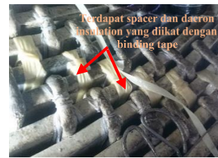
Figure 3.3 New Ties Addition
