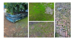
**Fig 2.** Clockwise from Left - Experimental Sample Vs Controlled Sample, Integration of moss and vegetation in crevices of brick pavers, Cracked and loosely packed brick pavers enabling more vegetal growth (Source: Aswin Senthil 2022)
